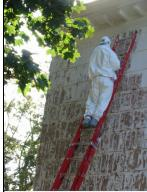
Wet scraping/ stabilization (removal of loose and flaking paint) performed by a licensed deleading contractor
