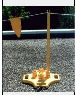
A roof boundary system is used to limit employees access to the fall hazard. The system includes posts, rope and warning flags distributed along the rope..
