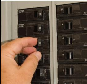
Locate the correct energy isolating device
