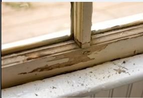
Flaking paint on a window sill—assume it contains lead paint unless testing indicates otherwise
