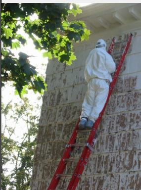
Wet scraping/ stabilization (removal of loose and flaking paint) performed by a licensed deleading contractor
